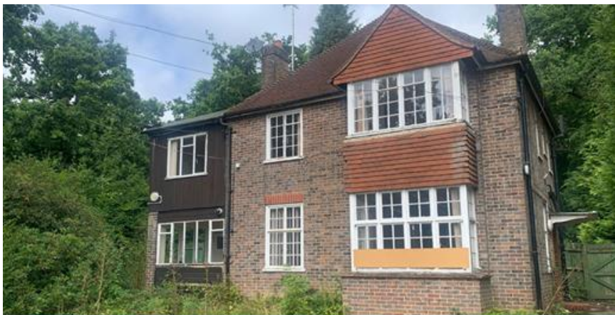
Fig.2 The House in the Wood residence to the north of St Piers Lane
